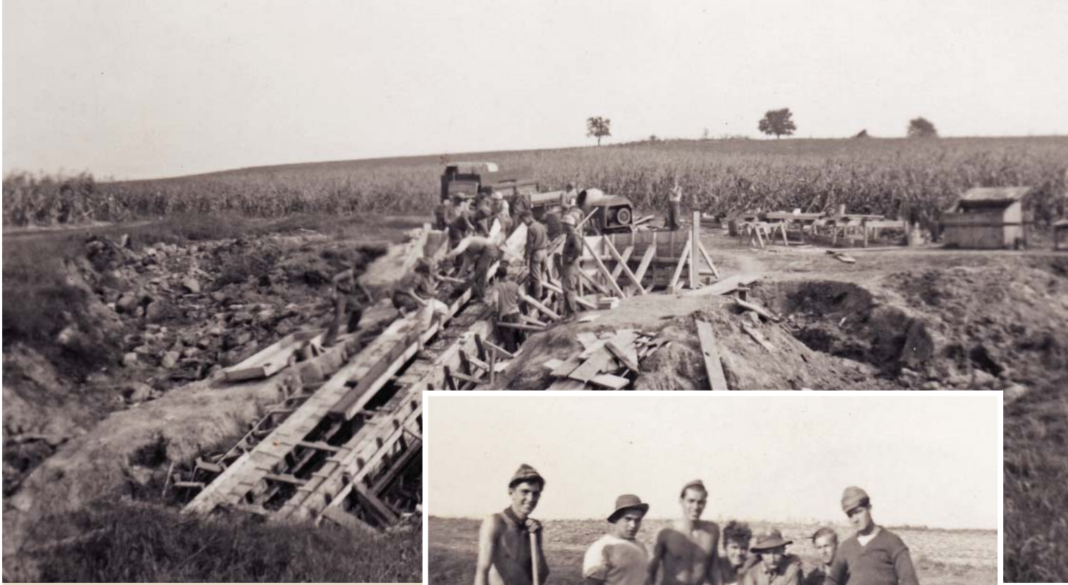
Spillway under construction, do you recognize any of the trees on the horizon?
