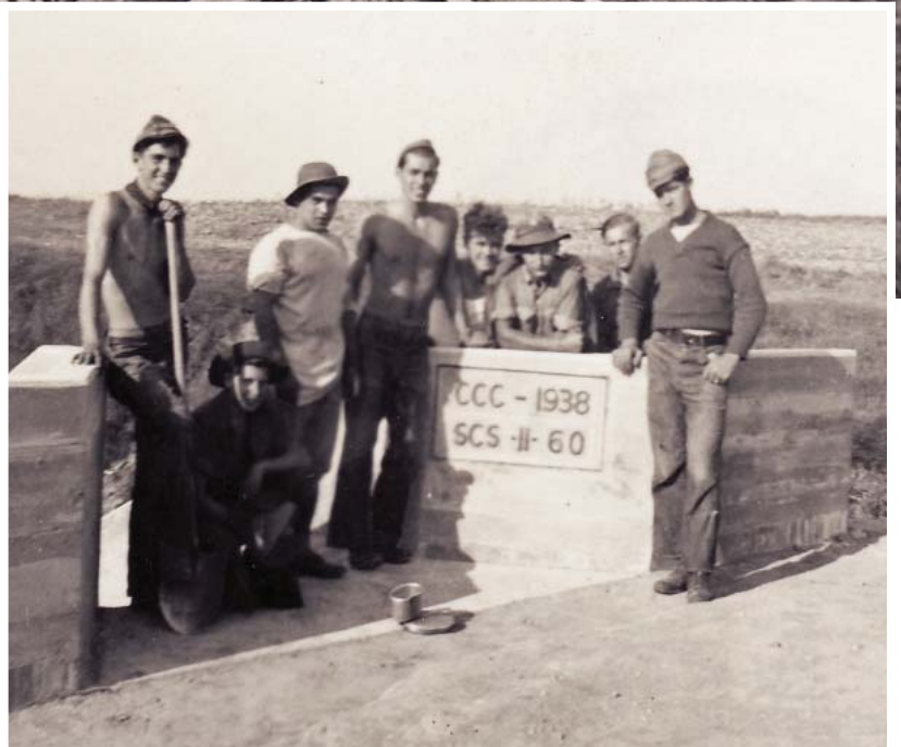
CCC boys 1938, notice the earth berms are not yet built off the wings of concrete.
