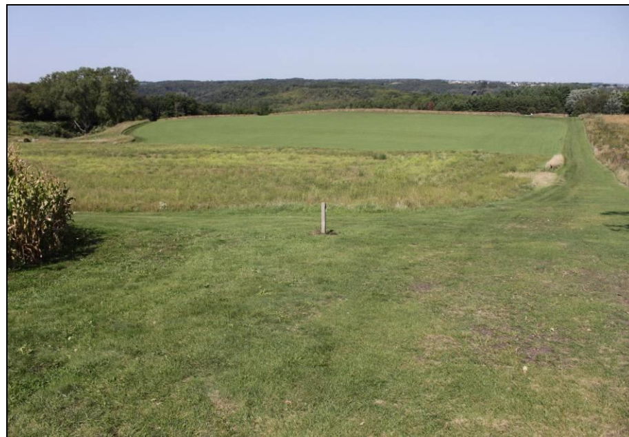
Looking downhill at second recessional moraine and CCC culvert on the left side of the photo.
