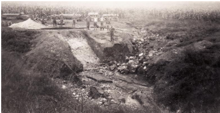
Pictured Left: CCC Spillway in 1938 (today the spillway is located at the PFC and is still functional)
