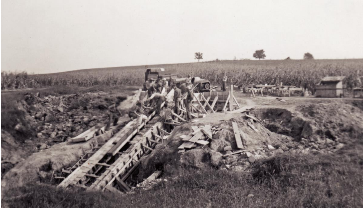
Above: Construction of the CCC Spillway at Pope Farm Conservancy
