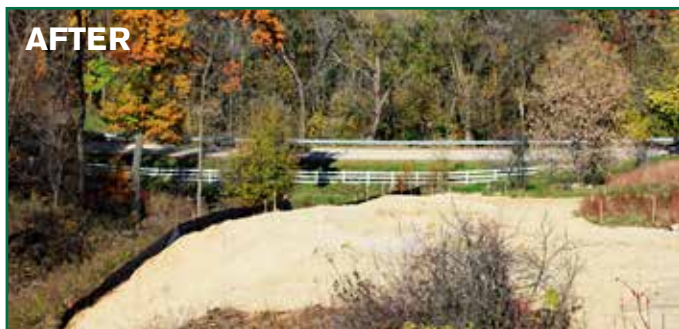
Black siltation fence is shown in the photo above on the left.
