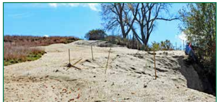
Repaired slope and relocated trail with biodegradable matting.
