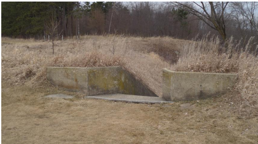
CCC Spillway at Pope Farm Conservancy Today
