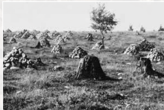
Clearing the Land—burnt stumps and stone piles
