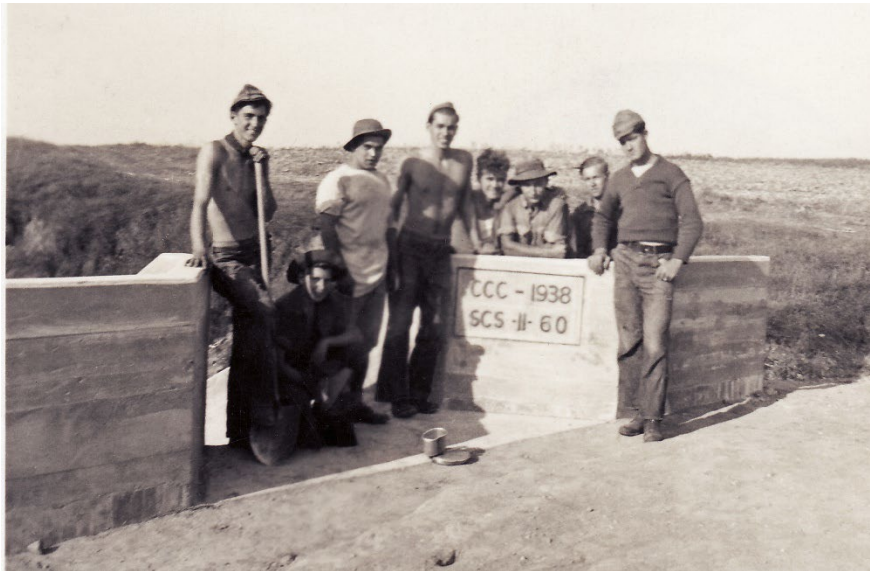
Above: CCC Spillway 1938
